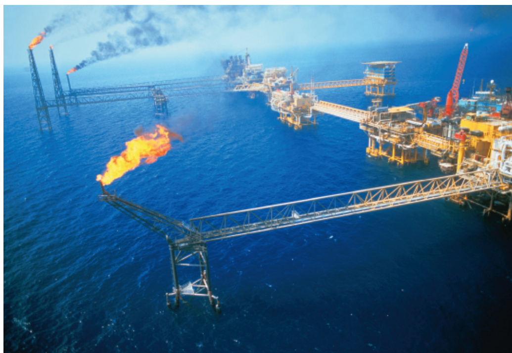
Figure 2 Offshore oil rigs, such as this one in the Gulf of Mexico, produce about one-fourth of the world's oil.
