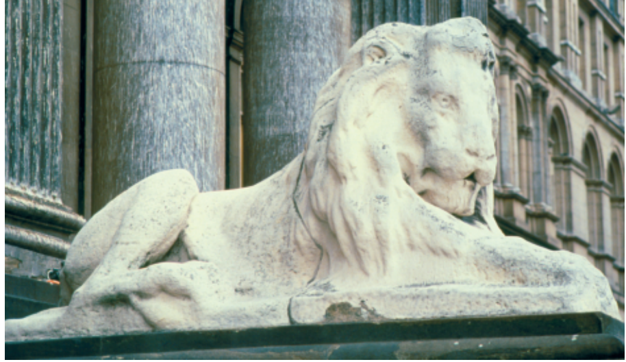
Figure 6 This stone lion sits outside Leeds Town Hall in England. It was damaged by acid precipitation.
